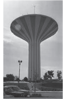
Water tower, Orebro.
